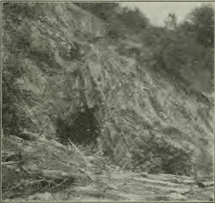
Photo No. 7. Tunnel at W. P. Thomas Manganese Mine, near Ukiah; Mendocino County. Orebody at this point above 4' wide.
